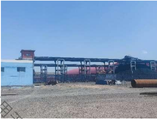
煤转运站及运煤通廊
